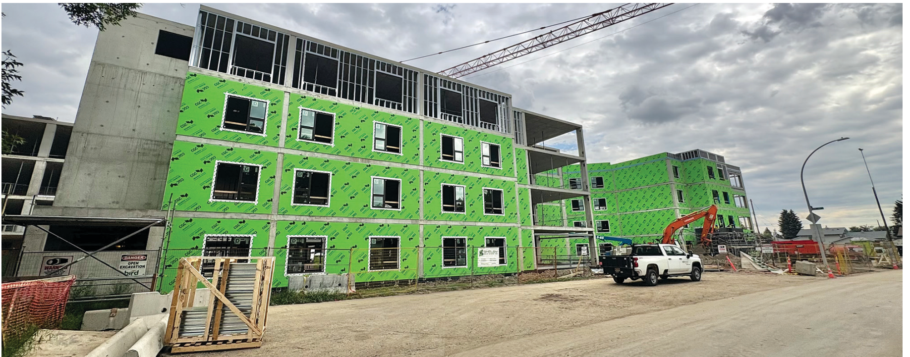
Above: Construction crews continue exterior work on the new school as masonry, windows and the main entrance begin to take shape. Below: Construction progresses on a multi-storey seniors' housing development as crews install windows and complete the building's exterior.
